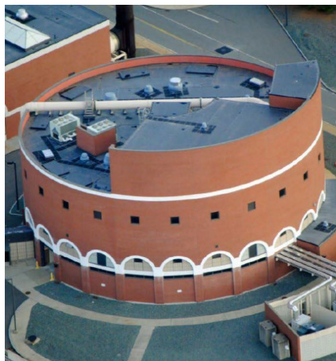
South System Pump Station
